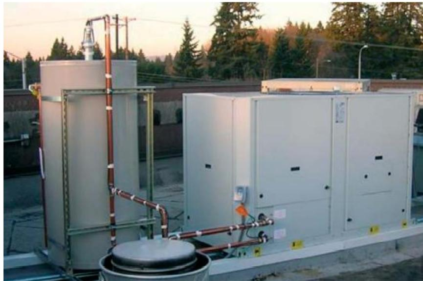
*Figure 3. Industrial 60kW CO<sub>2</sub> heat pump water heater (T. Seinel, IEA v.24.3.2006)*
